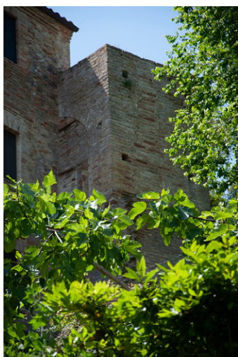
Fig. 7. The first tower of the western walls.
