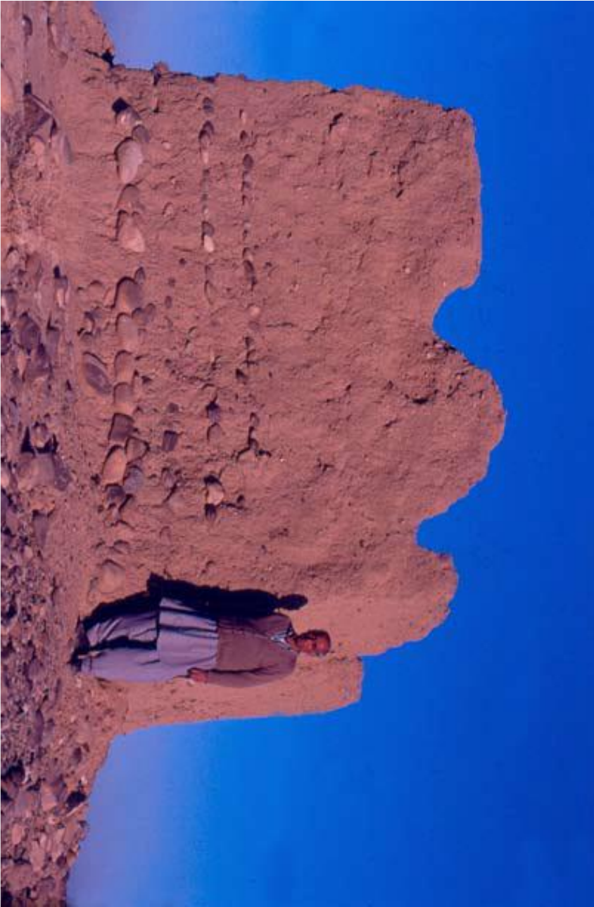
Fig. 4 - Prof. Farid Khan beside a recently abandoned structure in the west of Bannu District which shows the very effective traditional method of wall construction using boulders, cobbles and clay.
