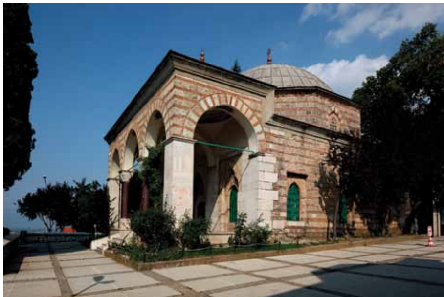
Figg. 14, 15. Bursa, türbe of Bayezid I, 1406
