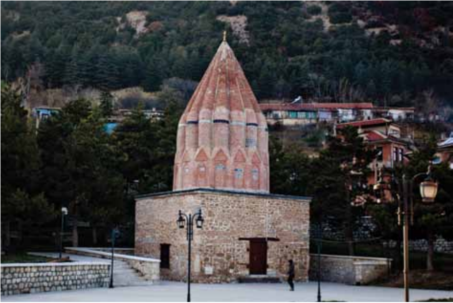
Fig. 13. Akşehir, türbe of Seyyid Mahmud Hayrani, 1224
