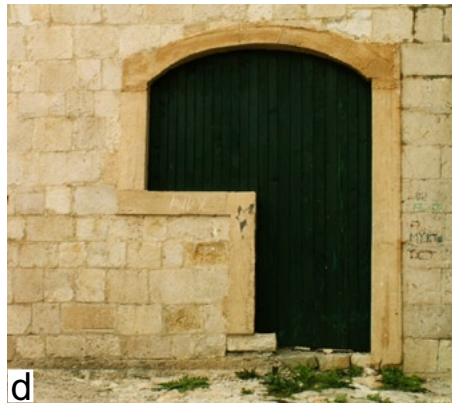
fig. 2.18 – Finestra in Stari Bar, UTCF 146b (a), Budva (b), Kotor (c), Ulcjni (d).
