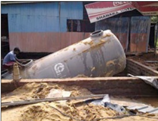
Figure 1: Eco-Tank being installed in Negombo in 2011
