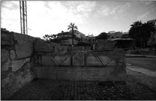
Figure 14. Photograph. Current view of the remaining walls conserved in the Basilica Thermarum. Detail of the paintings. Photograph coming from the archive of the project.
