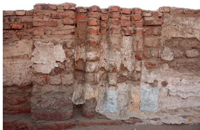
Figure 5. The painted composite buttress near to the western entrance (2012 season).
