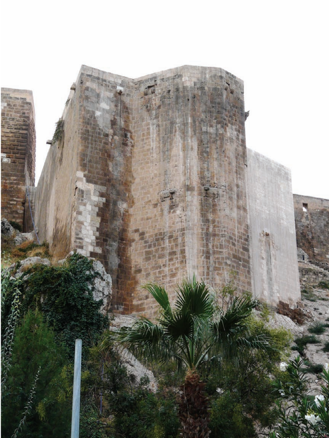
Fig. 9 – Rebuilding of the access system, from the North (Period 5, tower 4) (©C. Tonghini)
