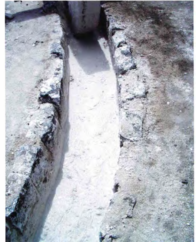
Lime mortar being crushed (AGTF Collection)
