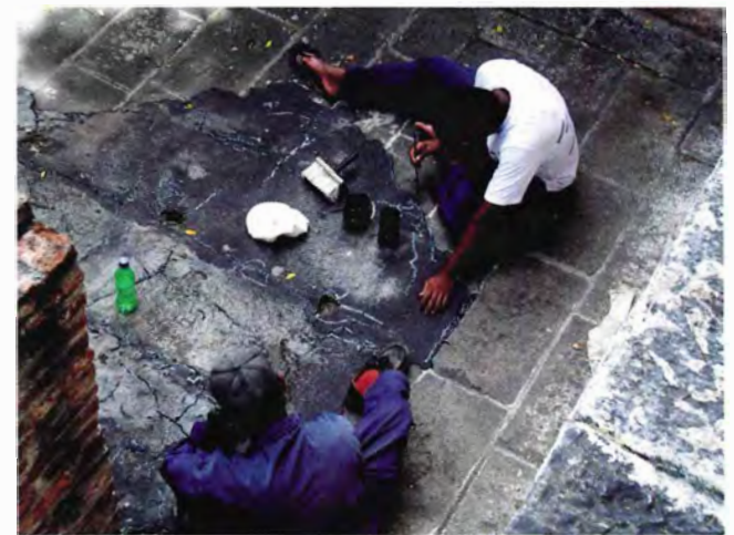
Consolidation of original tarfelt in privies area (AGTF Collection)
