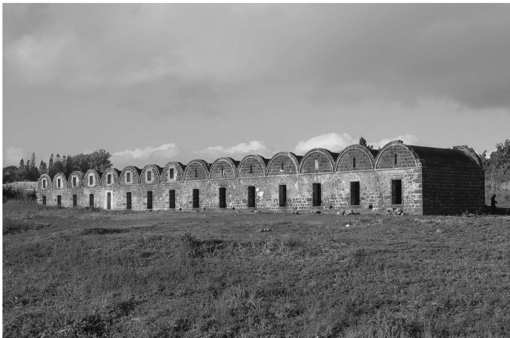
Fig. 2: Trianon Barracks, view from North
