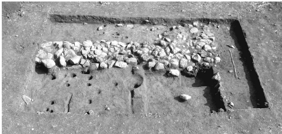
Fig. 10: SU 05, Foundation of the side wall of Structure A, view from North-East
