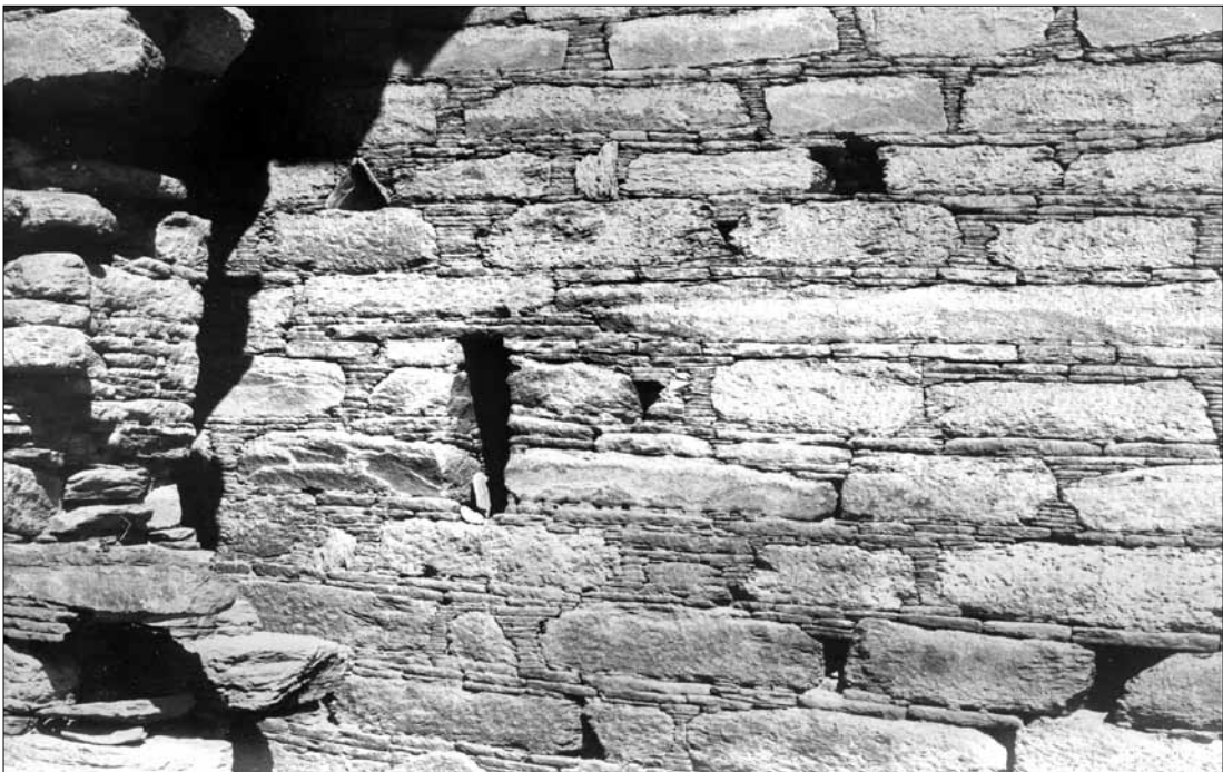
Fig. 479. Vihara of Gumbat. S corridor, N wall; aperture used for daylight and, above, triangular niche for oil-lamp. (Taddei 1959; Neg. CS).
