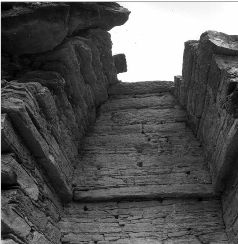
Fig. 509. Kanjar-Kote. Double vihara. E cell, pavilion vault. (Bonardi Tucci 1959; Neg. CS).
