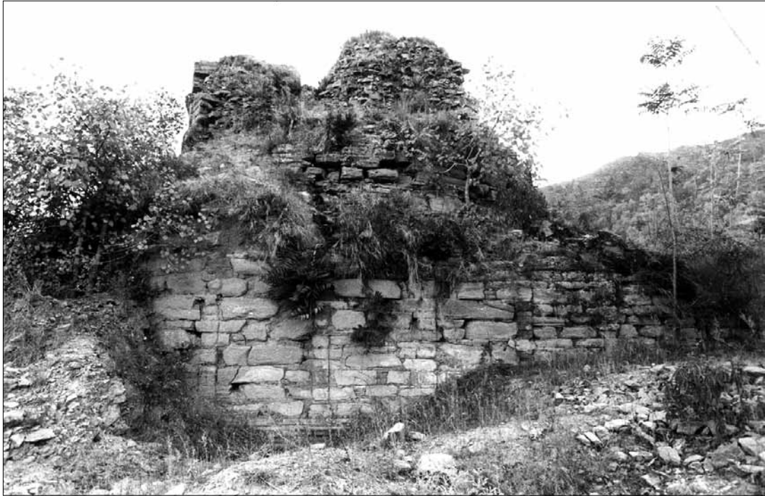
Fig. 28. Stupa of Jurjurai. General view, W side. (Nascari 1993; Neg. CS).
