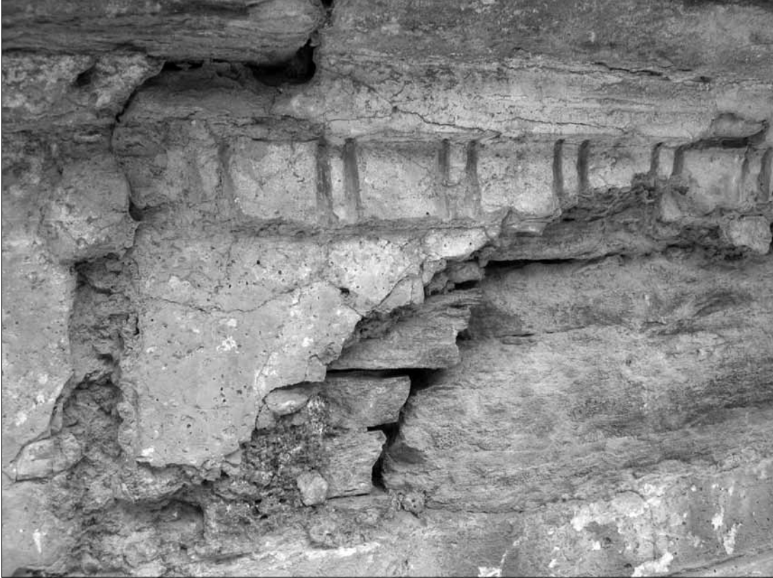
Fig. 303. Abbasahbchina. Stupa C. SE side, 3 rd storey; modillions of pilasters, stretch of architraved and bracketed cornice; plaster remains. (Spagnesi 2005).
