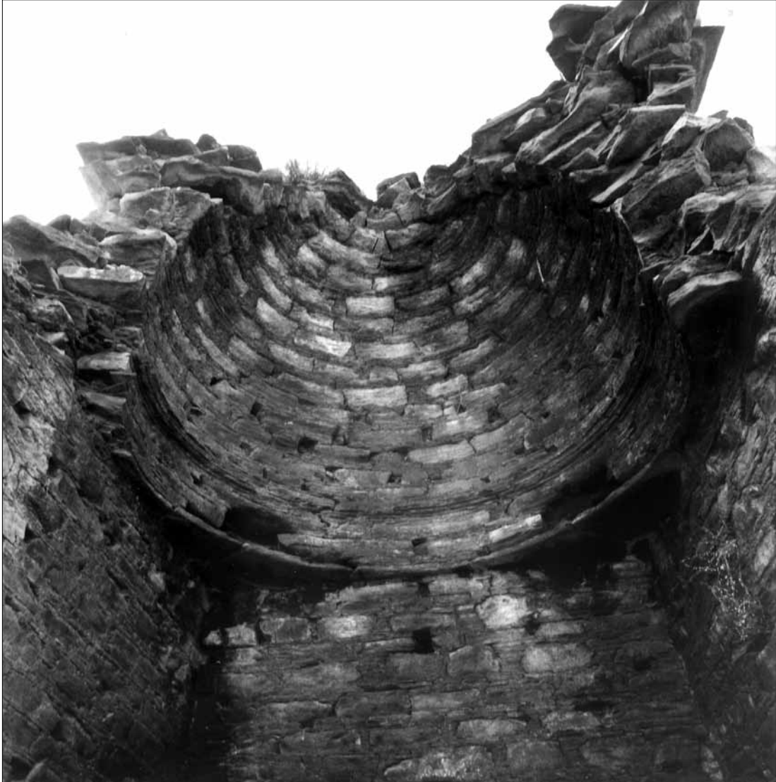
Fig. 446. Abbashechina, vihara F Inside of the aedicula (B); lower dome with springer on corner slabs and overlying band (F, G). (Kuwayama 1993).
