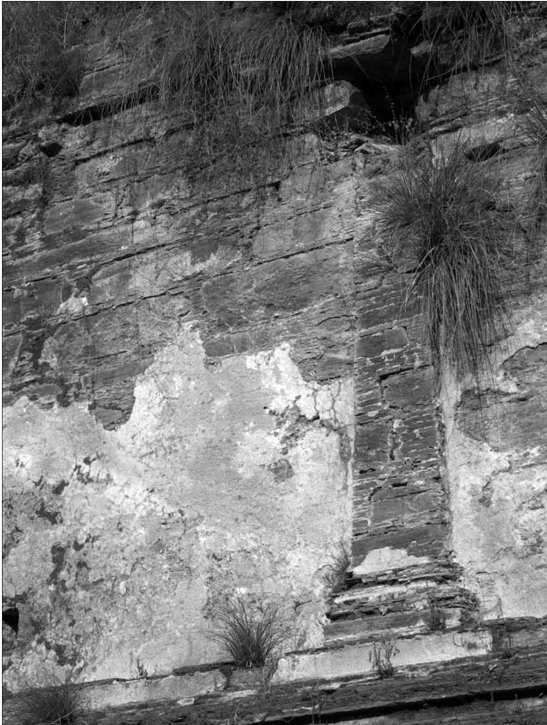
Fig. 288. Abbasahebchina. Stupa C. E side, 1 st storey, N stretch; detail of plaster remains. (Spagnesi 2005).
