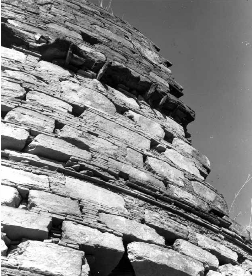
Fig. 422. Stupa of Gumbatuna. SE side; 3 rd storey (drum), 4 th storey (transition storey of the composite dome) with cornices. (Bonardi Tucci 1966; Neg. CS).
