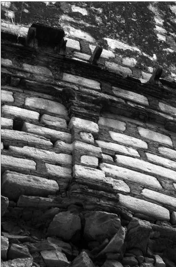
Fig. 146. Stupa of Shankardar. W side; 3 rd storey (drum) with pilasters, cornice with architrave and brackets; above the 4 th transition storey of the raised dome. (Sabelli 1993).
