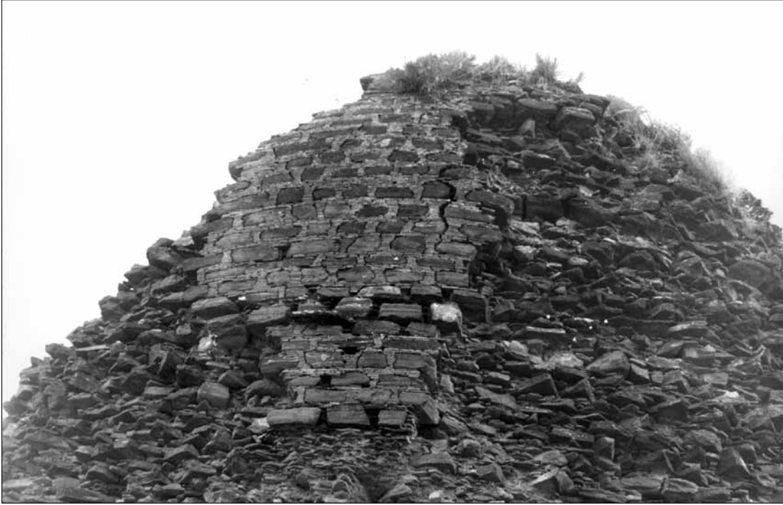
Fig. 380. Barikot, Stupa A. NE side, with a short stretch of the preserved facing; belonging to the upper part of the transition storey of the composite dome and to the lower part of the same dome raised with projecting slab; elevation. (Scerrato 1959; Neg. CS).
