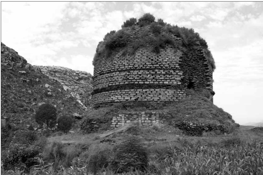
Fig. 174. Stupa of Amluk Dara. General view of the NE side. (Spagnesi 2005).
