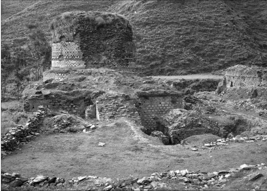
Fig. 337. Stupa of Tokar Dara (Najigram). W side with the stairway. (Spagnesi 2005).
