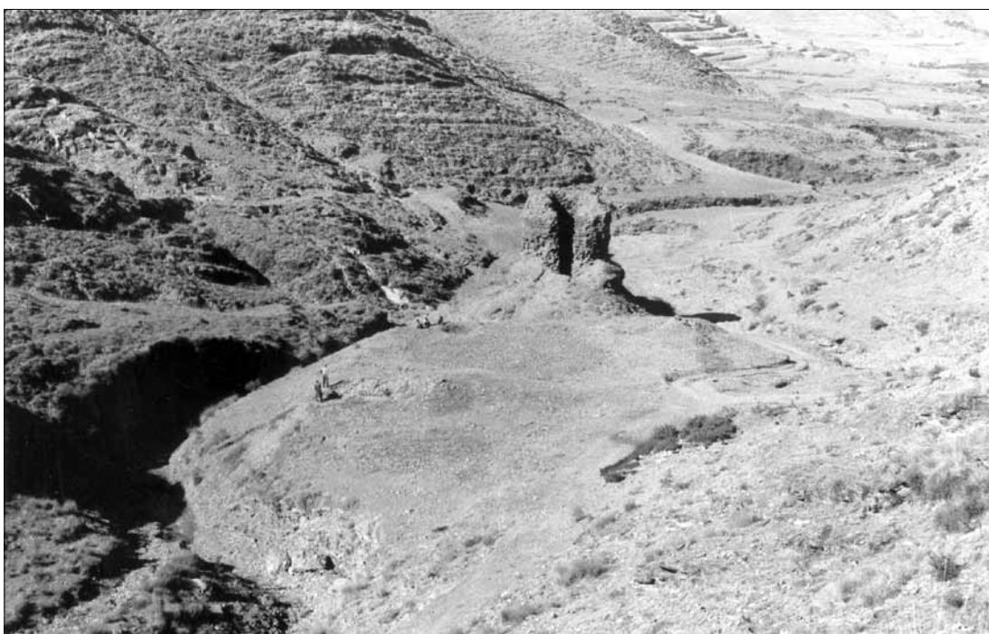
Fig. 398. Stupa of Top Dara (Haibatgram, Thana). E side; general view showing the cut through the stupa core; the quadrangular structure of the monastery looms in the foreground. (Sabelli 1993).
