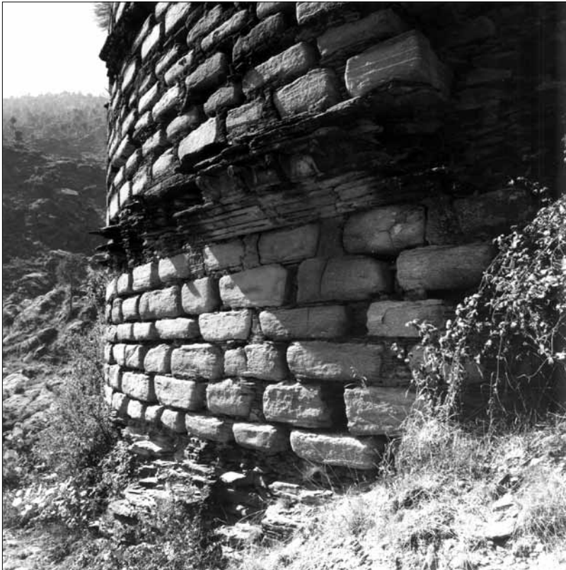
Fig. 181. Stupa of Amluk Dara. 3 rd storey (drum) with base (missing) and cornice with brackets (four of them have been conserved) and 4 th transition storey of the composite dome. (Kuwayama 1993).
