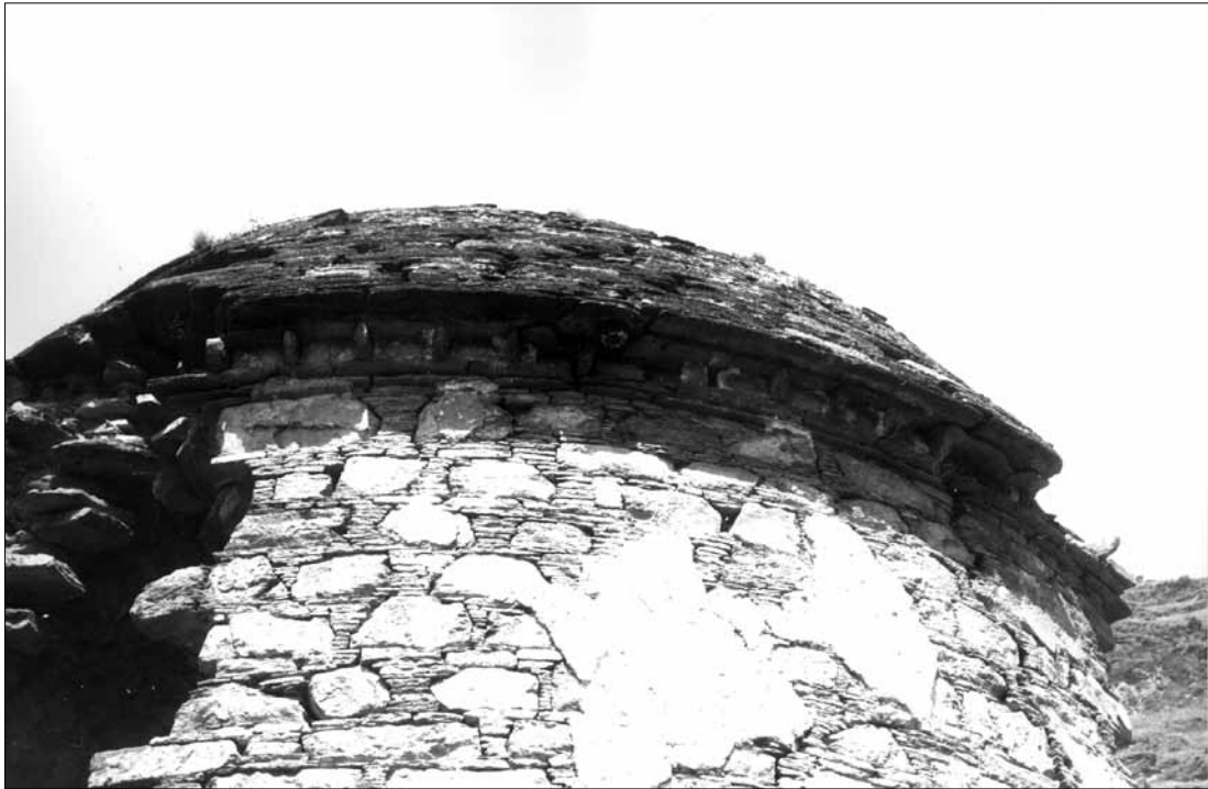
Fig. 520. Gumbatuna, Vihara. SE side; upper part of the outer wall of the cell showing remains of plaster, cornice and the beginning of the dome. (Faccenna 1960; Neg. CS).
