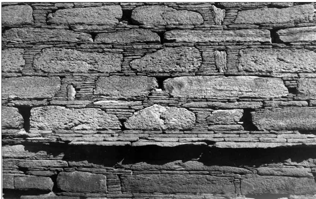
Fig. 470. Vihara of Gumbat. S side; detail of the decoration of the podium and of the construction technique. (Taddei 1959; Neg. CS).
