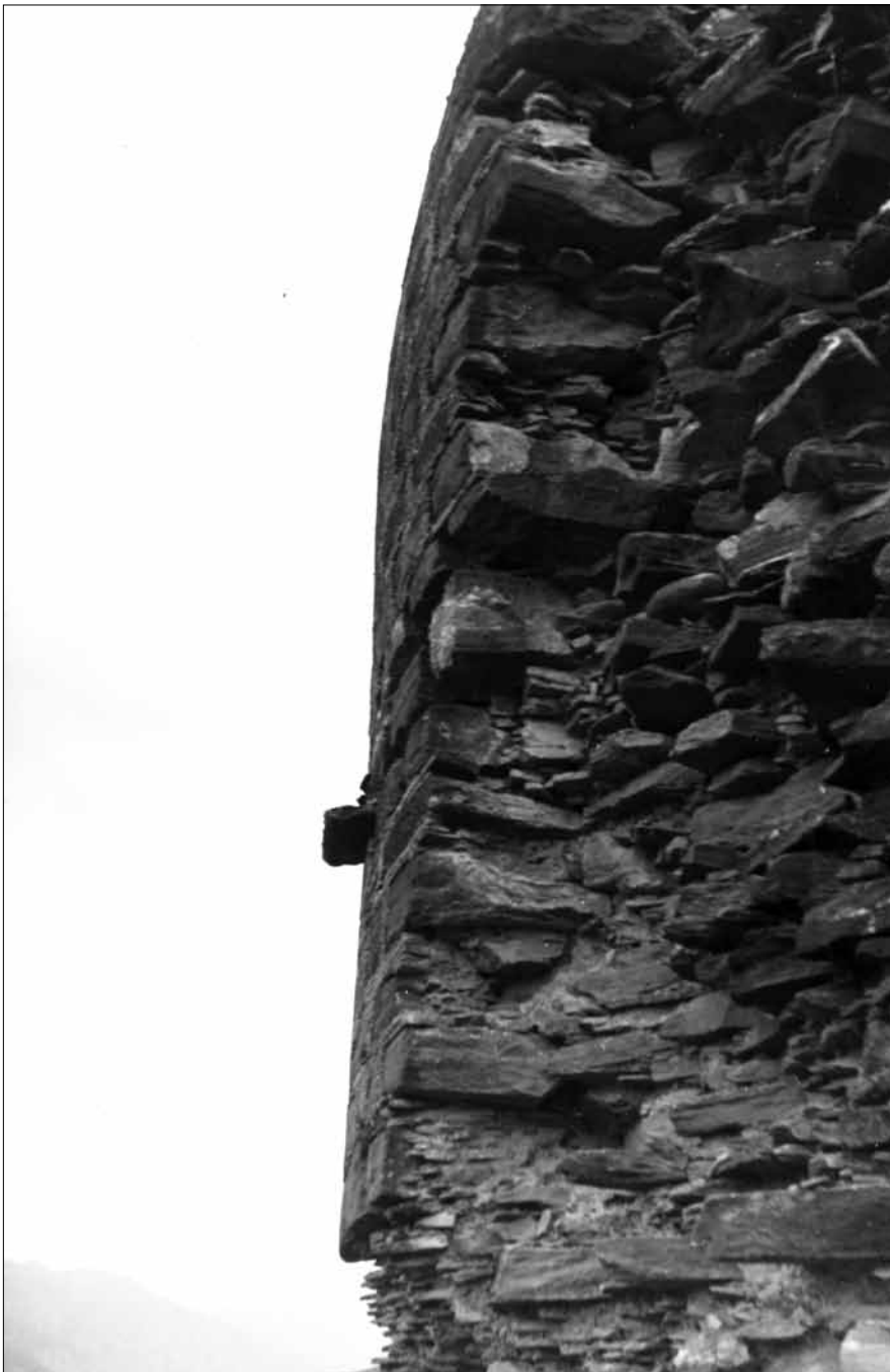
Fig. 381. Barikot, Stupa A, profile showing the projecting slab of the dome. (Scerrato 1959; Neg. CS).
