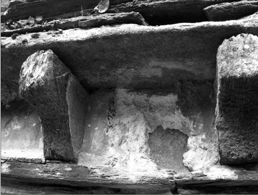
Fig. 183. Stupa of Amluk Dara. 3 rd storey (drum), cornice; detail showing brackets and plaster. (Spagnesi 2005).
