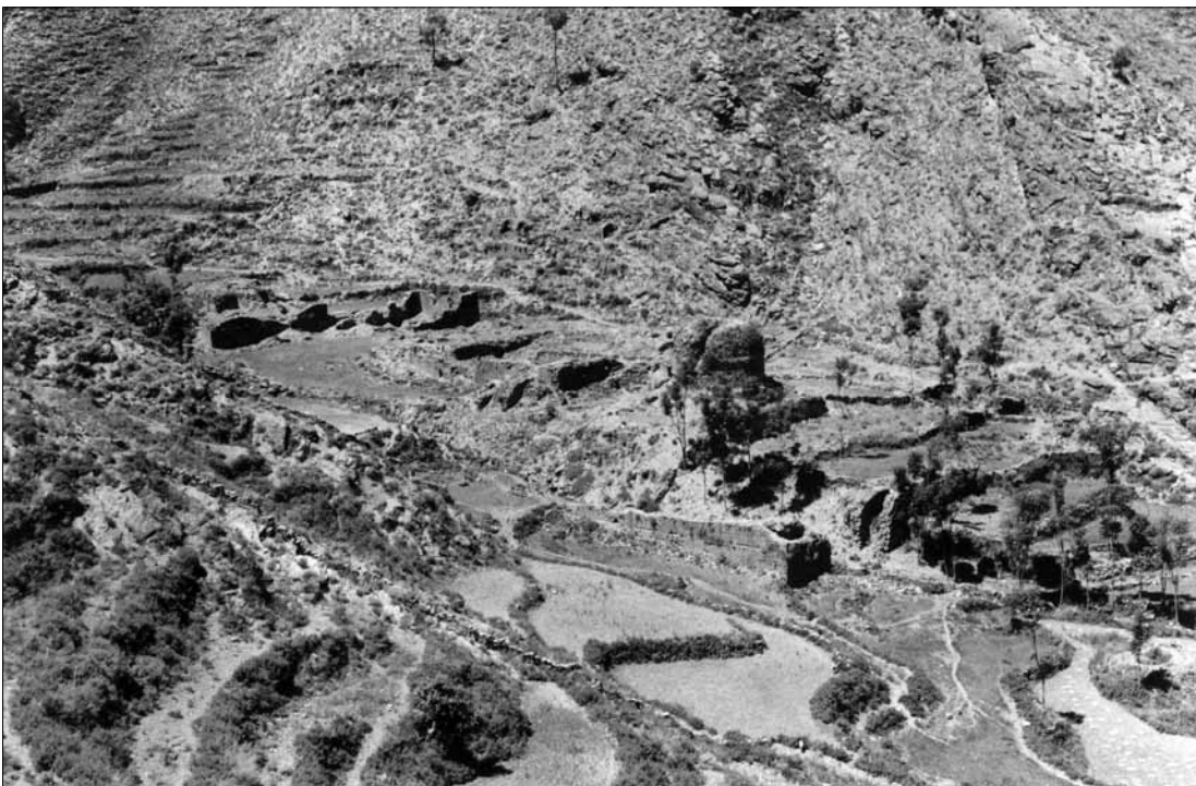
Fig. 331. Tokar Dara (Najigram). General view of the complex; from N to S; from right to left: aqueduct, stupa, monastery, vihara. (Spagnesi 2005).
