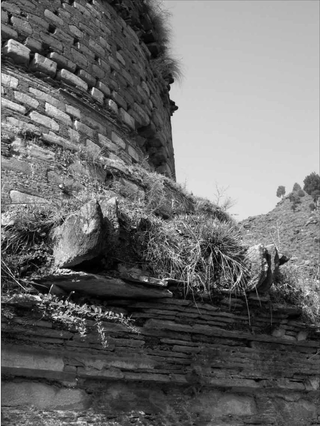
Fig. 350. Stupa of Tokar Dara (Najigram). N side, 1 st storey, cornice with brackets; detail. (Spagnesi 2005).
