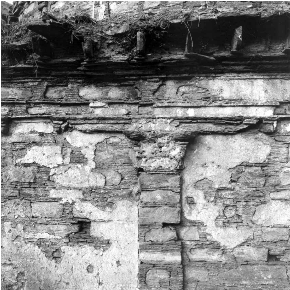
Fig. 233. Abbasahebchina. Stupa A. S side, 1 st storey, with remains of plaster. (Kuwayama 1993).
