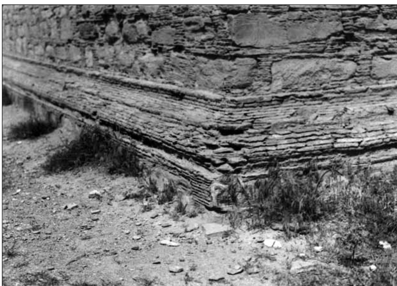
Fig. 419. Stupa of Gumbatuna. 1 st storey, corner moulding of the base. (Rockwell 1994; Neg. Cs).
