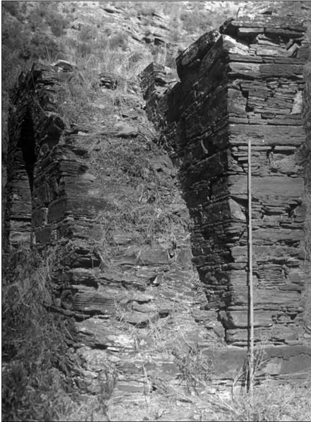
Fig. 528. Abbashehchina, dwelling unit. E side, stairway. (Faccenna 1957; Neg. CS).
