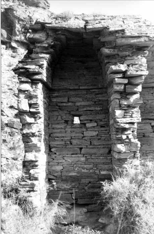
Fig. 506. Kanjar-Kote. Double vihara. S side (front); left cell (W). (Bonardi Tucci 1959; Neg. CS).
