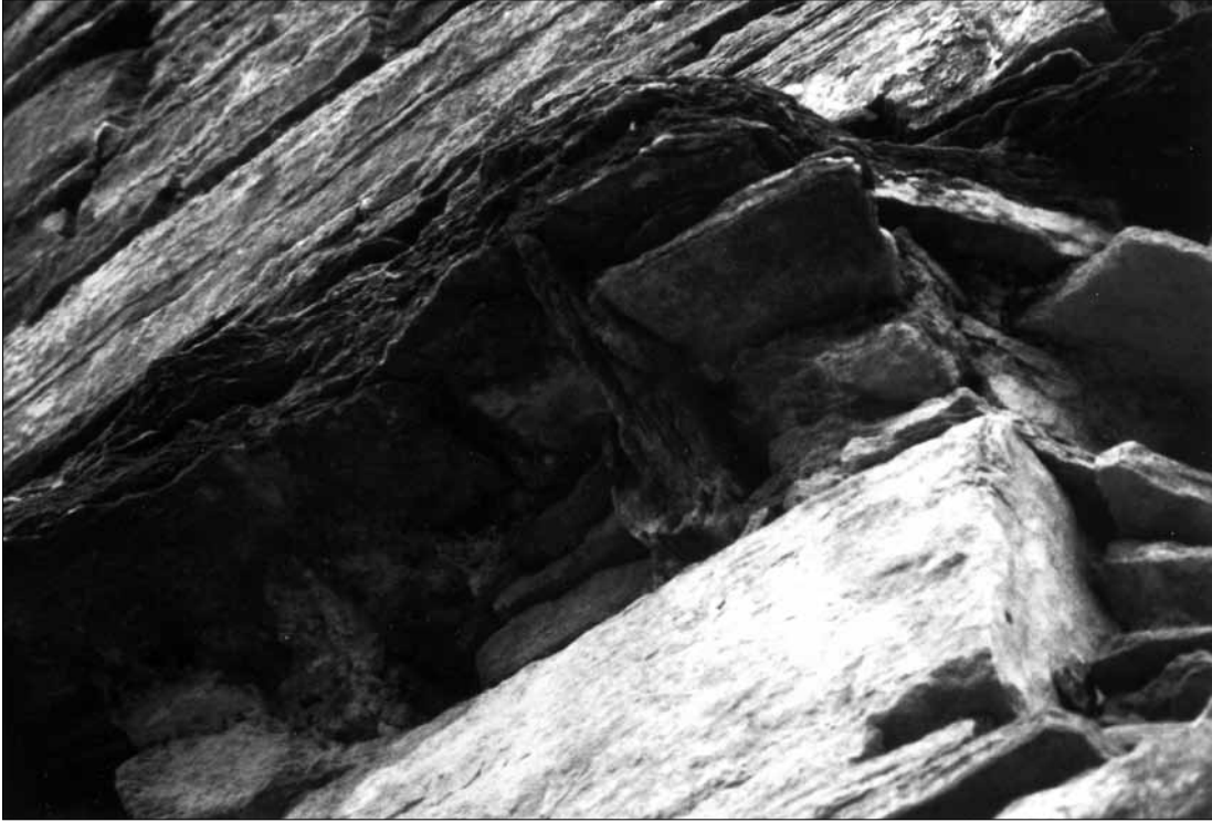
Fig. 424. Stupa of Gumbatuna. SE side; 4 th storey (transition storey of the composite dome) and cornice, detail. (Sabelli 1993; Neg. CS).
