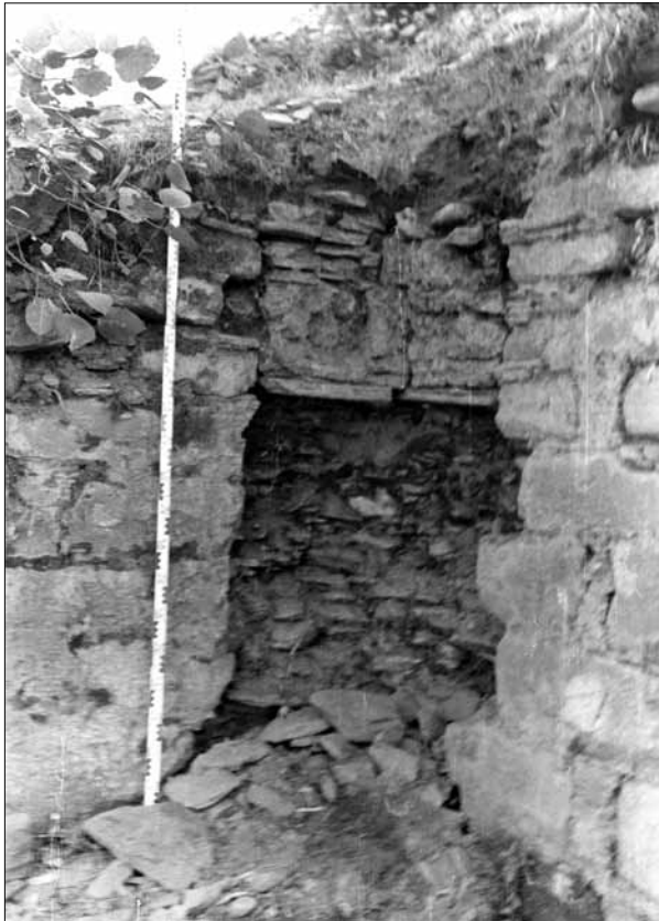
Fig. 177. Stupa of Amluk Dara. 1 st storey. N side. Stairway, E side, inner corner pilaster of the stairway and storey. (Sabelli 1993).
