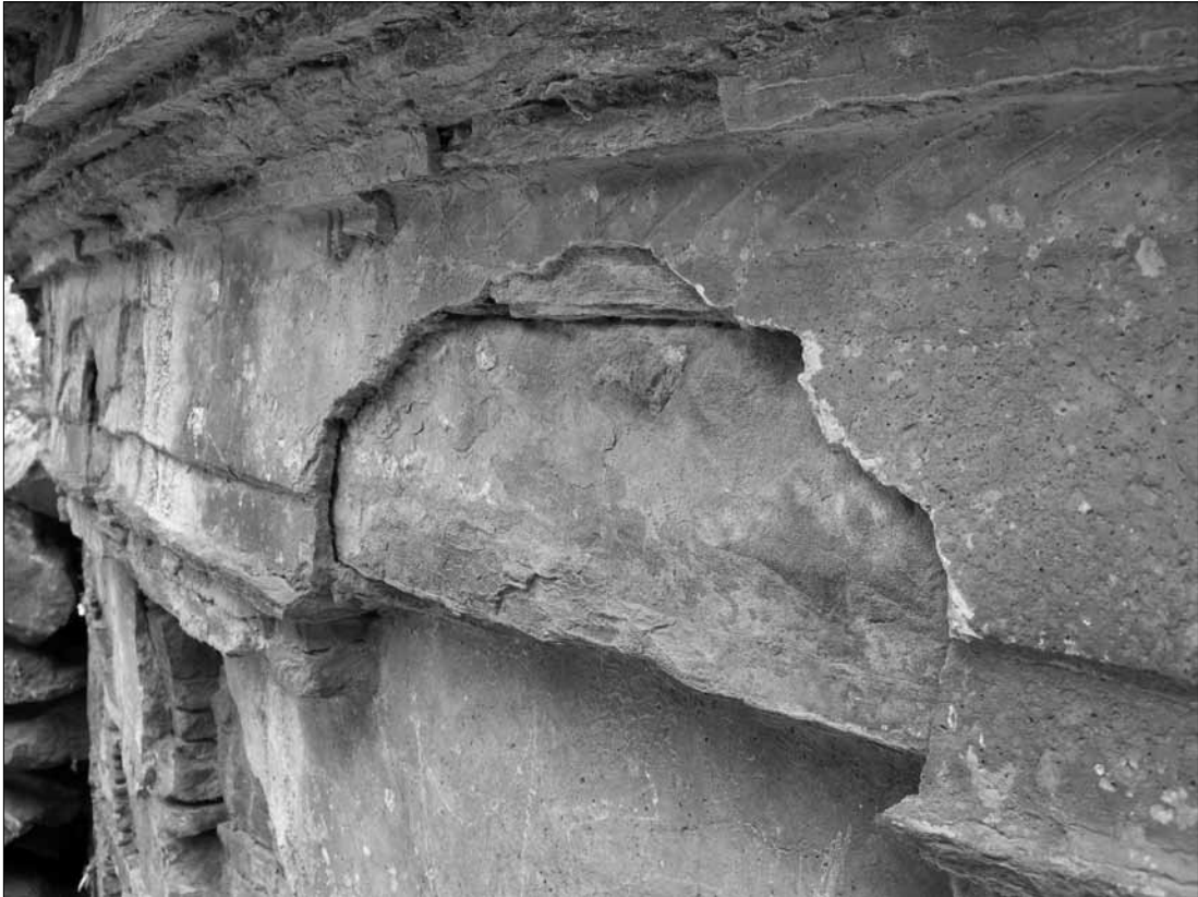
Fig. 301. Abbashehchina. Stupa C. SE side, 3 rd storey; modillions of pilasters, stretch of architraved and bracketed cornice; plaster remains. (Spagnesi 2005).
