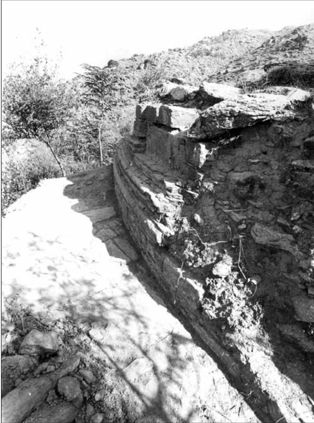
Fig. 56. Stupa of Loebanr. 2 nd storey, S side, with a stretch of the storey and floor; view from E. (Nascari 1991; Neg. CS).
