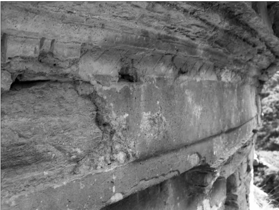
Fig. 304. Abbasahbchina. Stupa C, SE side, 3 rd storey; modillions of pilasters, stretch of architraved and bracketed cornice; plaster remains. (Spagnesi 2005).
