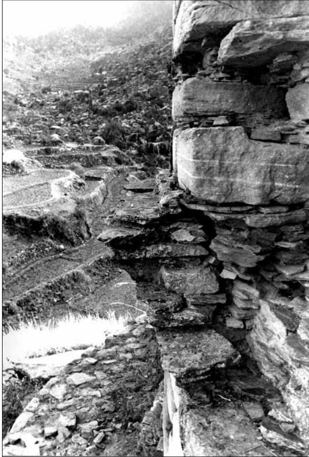
Fig. 184. Stupa of Amluk Dara. 3 rd storey (drum), cornice, view of the profile on the W. Above, springer of the 4 th transition storey, with projecting slabs. (Nascari 1993; Neg. CS).
