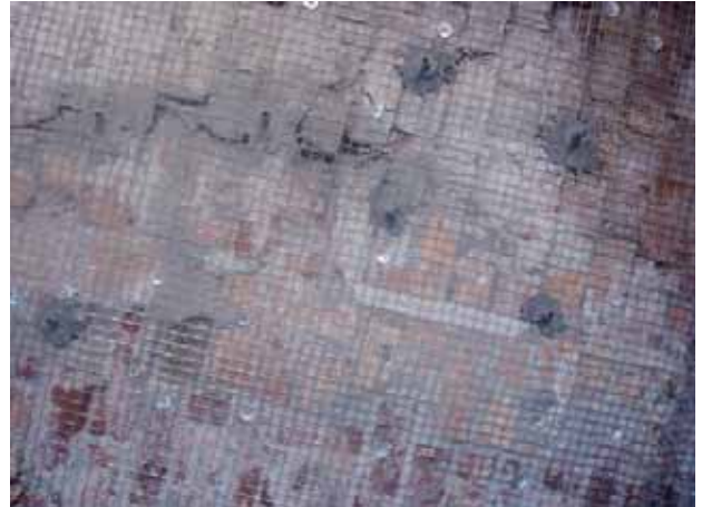
23. Wire mesh application and fixing injection nozzles
