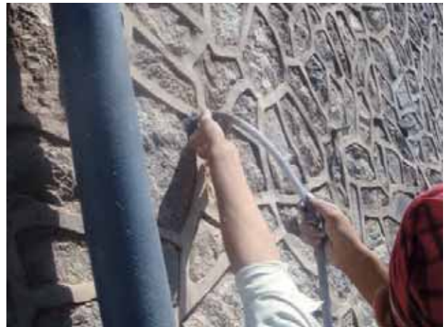
24. Stabilization of stone masonry façade by grout injection
