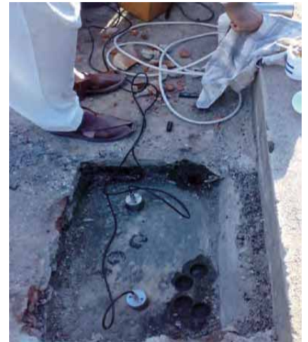
8. Ultra-sonic Pulse Velocity test in progress
