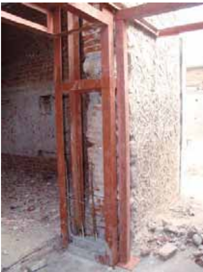
29. Steel reinforcement structure in the opening
