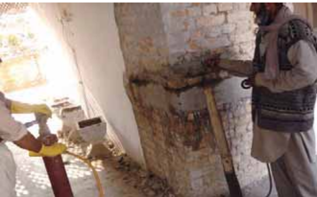
19. Cement based grout injection, Commerce College Mansehra
