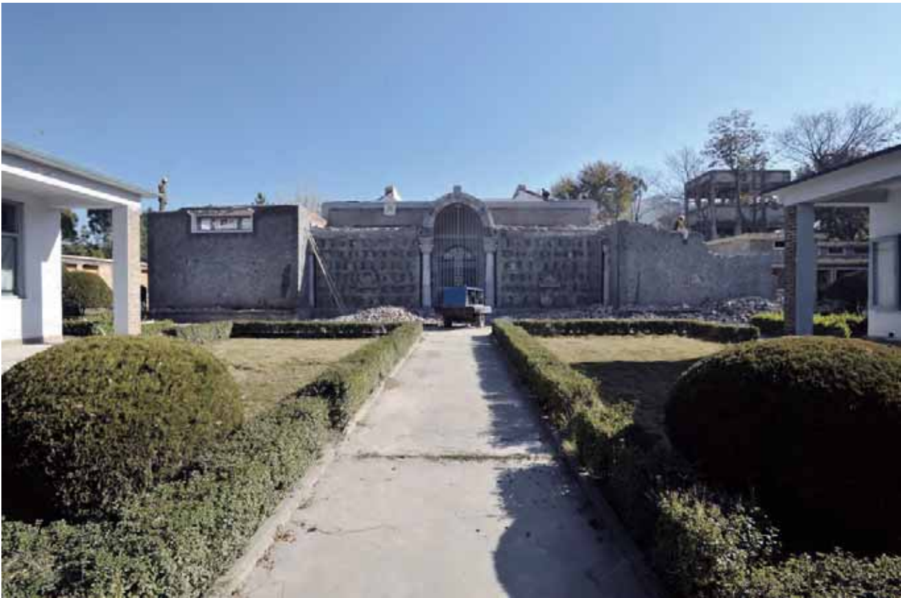
Old façade: Selective demolition (photo by E. Loliva)
