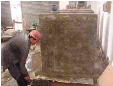
14. Application of ferrocement overlay
