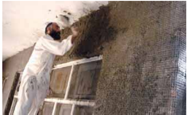
18. Application of ferrocement overlay, Commerce College Mansehra
