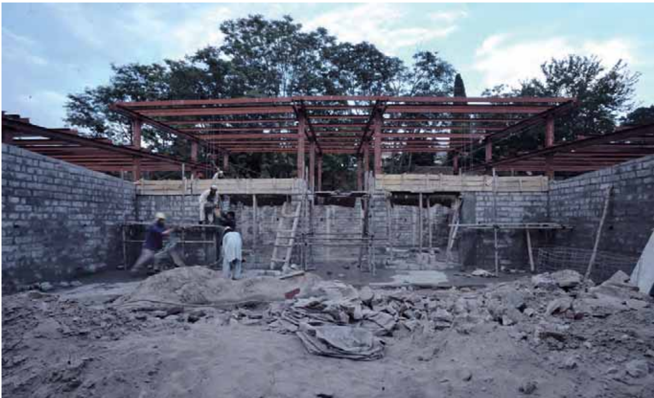
Block B: elevation structure (photo by E. Loliva)
