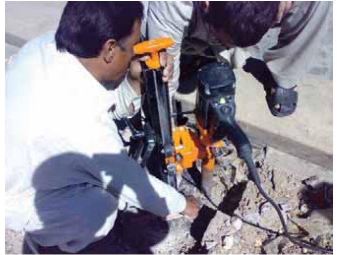
7. Core cutting in progress from roof slab
