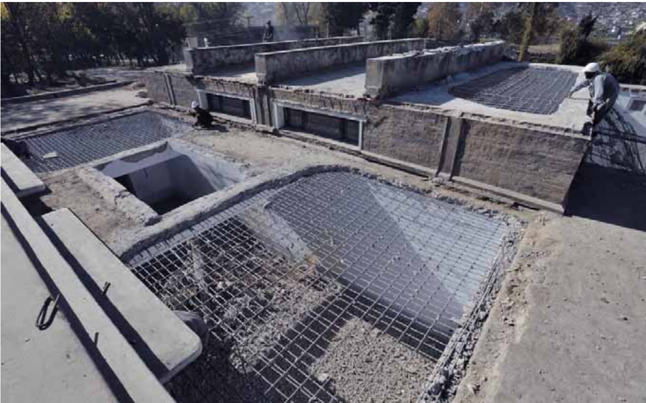
Block H: Selective demolition (photo by E. Loliva)
