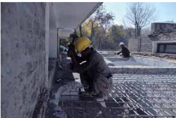
Block H: Selective demolition (photo by E. Loliva)
