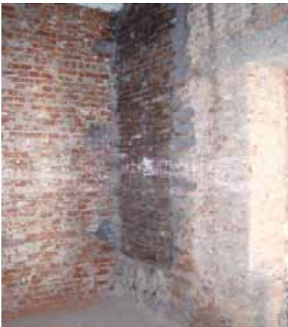
27-28. Reconstruction of corner wall
