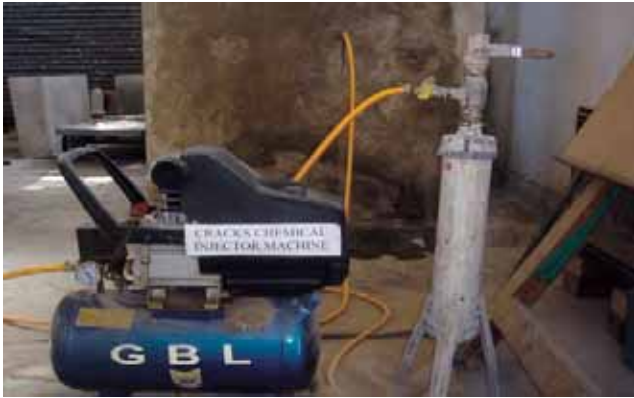
17. Grout injection in masonry wall
