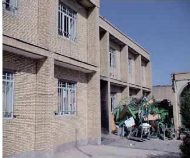
22. School building in Bam
