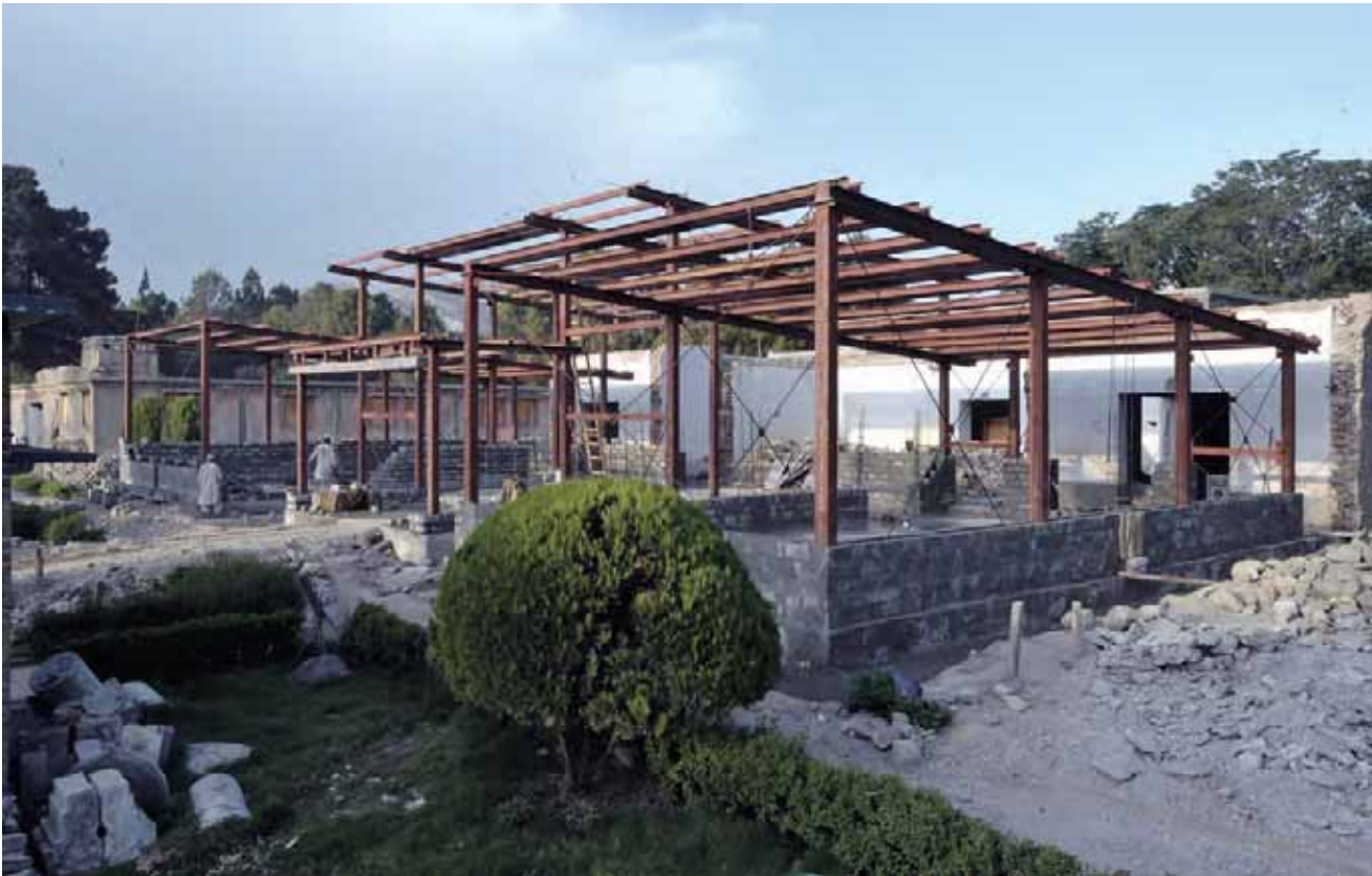
Block A: elevation structure (photo by E. Loliva)
