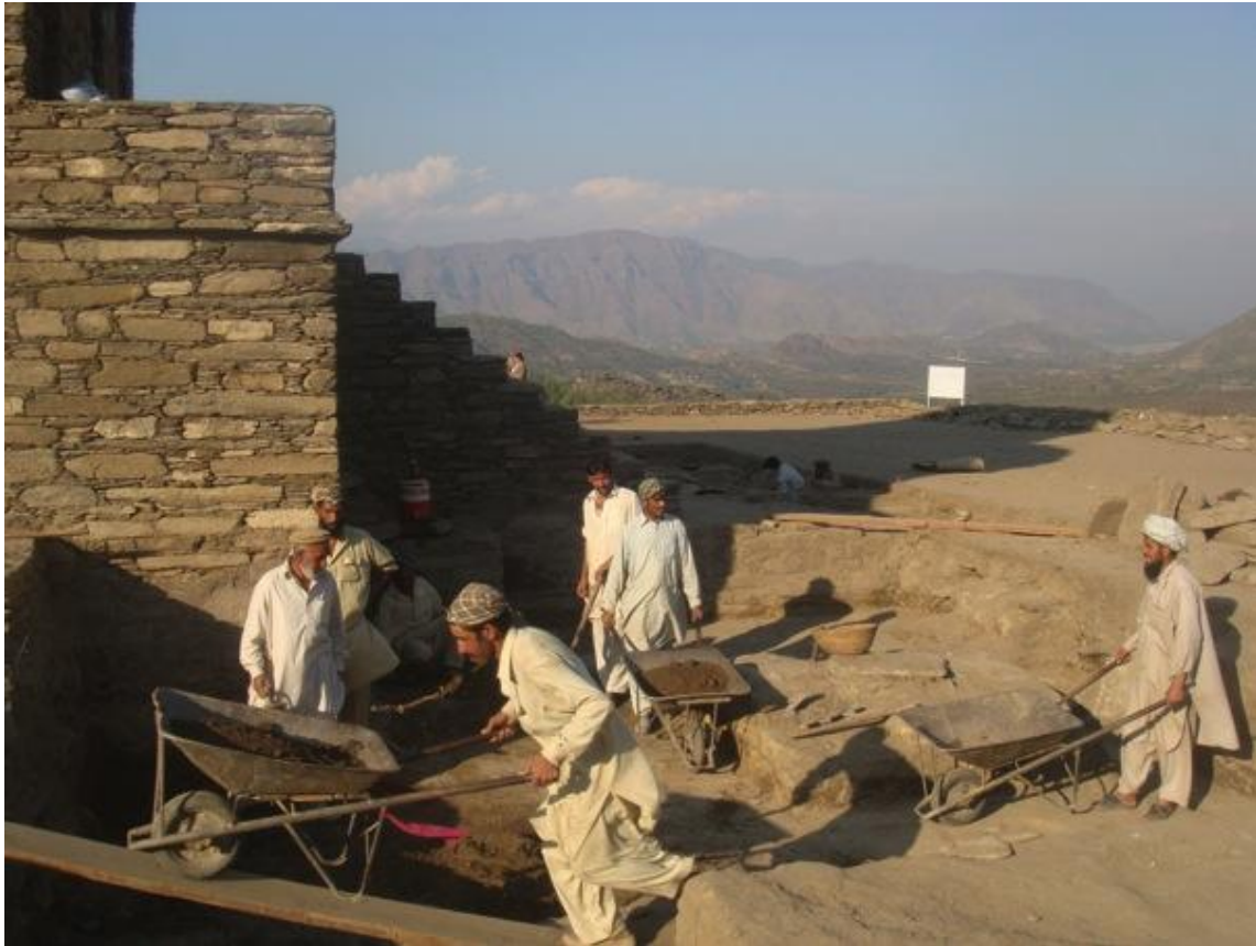
Figure 3: Excavation at Gumbat (Balo Kale) photo by E. Loliva, courtesy ACT
