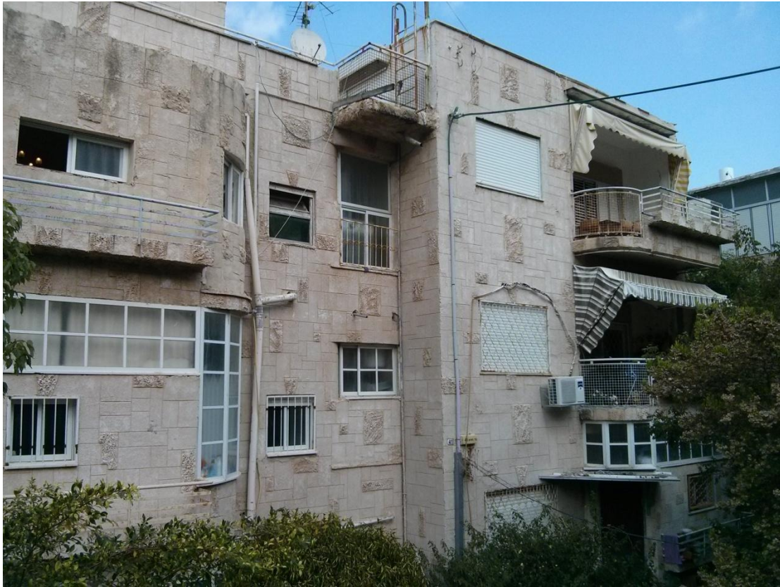
Figure 5: Theodor Menkes, Abramson building, Hadar, 1938 (Recent renovation, Covered with fake stone) ©Tzafrir Fainholtz
