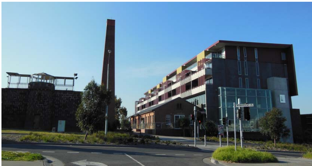
Figure 7: Former Boiler House and adjacent modern apartment block
