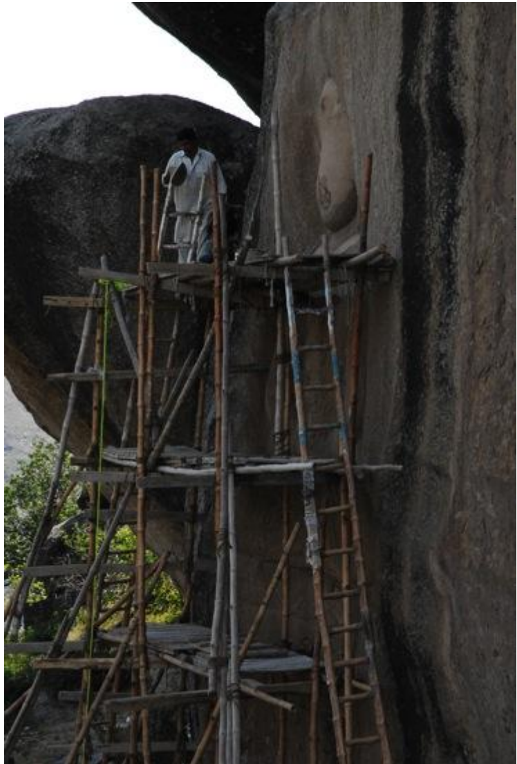
Figure 5 : Restoration phase at Jahanabad
