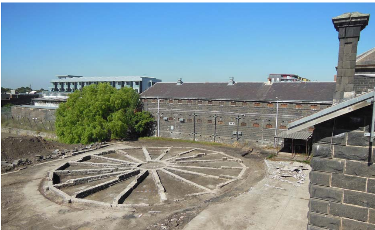
Figure 12: Excavated A Division panopticon exercise yard showing Foundary conversion and modern apartment block to rear ©Sarah van der Linde 2014
