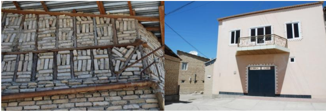
Figure 3: Traditional adobe brick with wooden frame building structure (left) and new construction within the historic centre (right) © Bukhara UNESCO GIS Project
