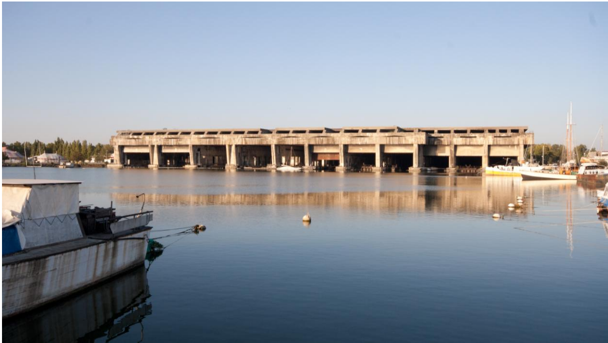
Figure 2: Photo of the Submarine Bunker in Bordeaux © Benjamin Schmidt
