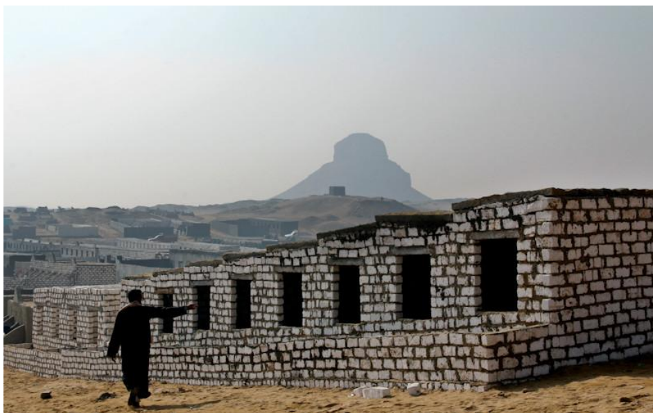
Figure 20: inhabitants of Dahshur proceeding to build new cemeteries in the absence of security forces ( photo: Roger Anis photographer )
