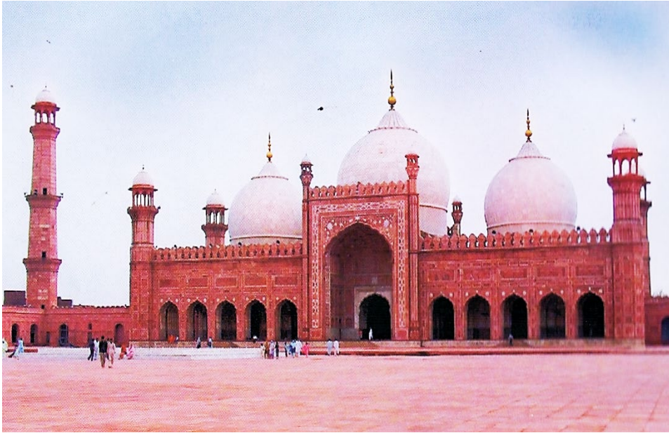
Fig.3 General view of Badshahi Masjid from the east (photo by the present researcher)
