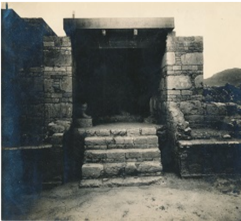
Plate-O: This 278 mm x 200 mm black and white monochrome photograph of Dharmarajika stupa, Taxila after repairs, of chapel N17. Steps lead up to the repaired chapel, which has a new roof.
