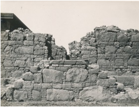
Plate-E1: This 203 mm x 135 mm black and white monochrome photograph depicts detailed view of the east face of the steps leading to the courtyard of what has been termed the later monastery. In the background, to the left of the image, a modern shelter is visible.
