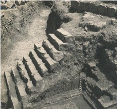
Plate-M: This 200 mm x 134 mm black and white monochrome photograph of Dharmarajika stupa showing detail of the north steps of the main stupa (Christope), from the north-west.
