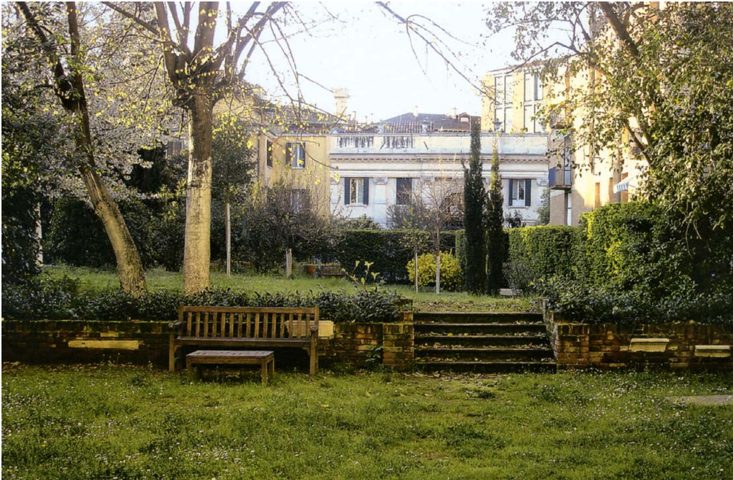
12. Venice, Casino library of Palazzo Foscari, mid-seventeenth century, view from the garden of Palazzo Vendramin.
