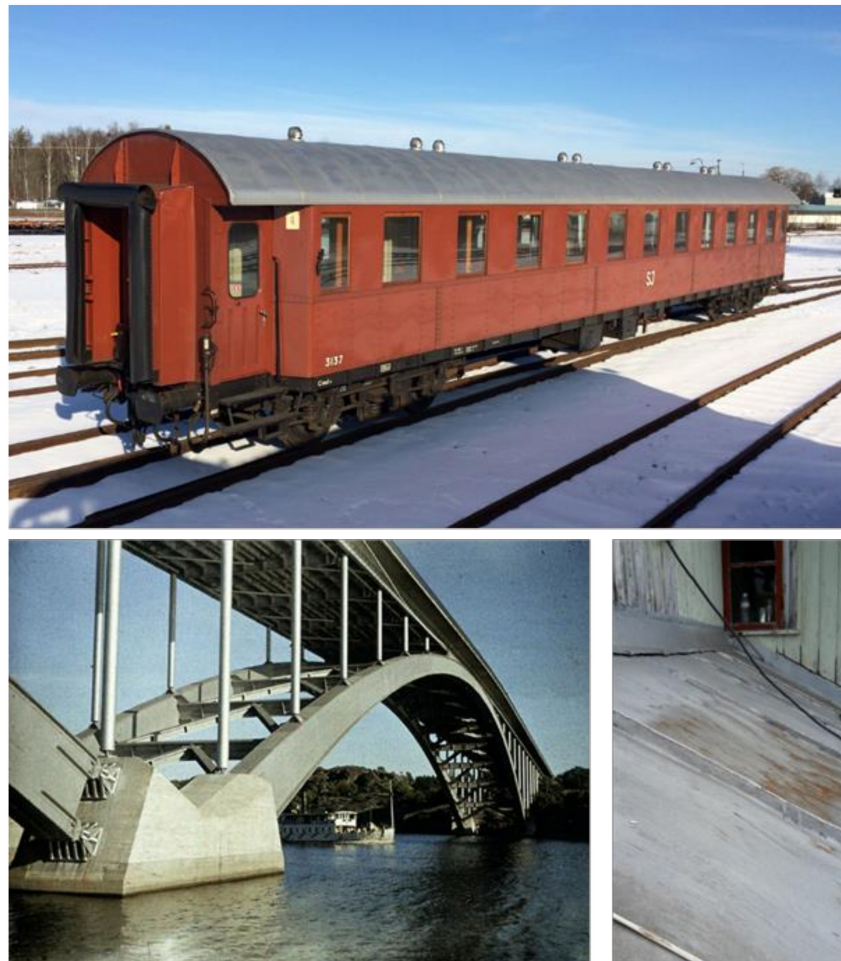
Figure 1. Examples of armour paint on historical ferrous structures. Top: A train wagon from 1936 with armour paint roof. Photo: Anna Lindgren 2019. Left: Västerbron in Stockholm, painted with amour paint in 1936. Photo: Cronquist, Gustaf W:son, unknown year (CC-BY). Right: Steel sheet roofing in 2019, last time repainted with armour paint in the 1960s (without primer). Photo: Tom Granath 2019.
