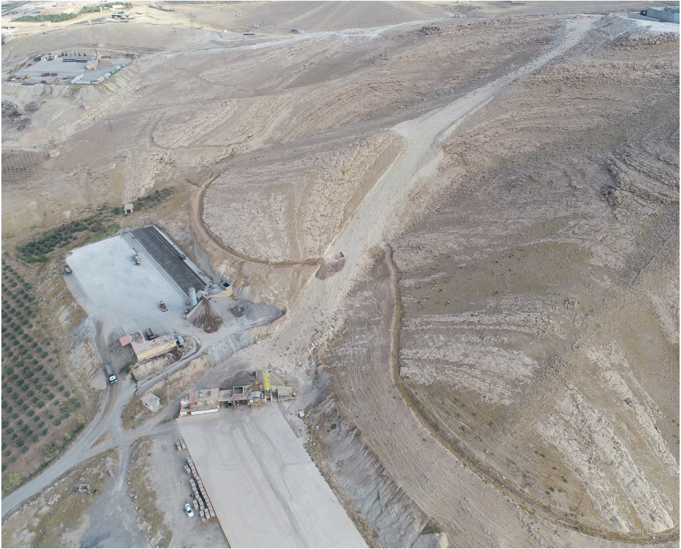
Figure 9 Drone view of three of the four concrete block factories built close to the Assyrian canal at Faida. Note the new aqueduct built in 2018 (top right) and the large trench for housing the water pipe that cuts the canal in two (photography A. Savioli)
